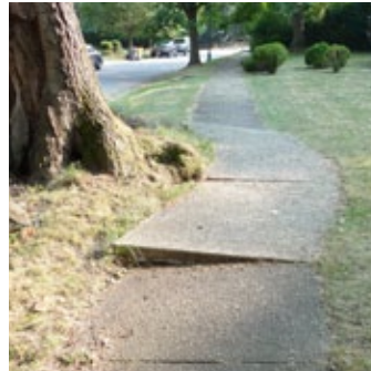
Take note of the Guilford sidewalk areas that may have been damaged due to a City-owned tree(s) located in the easement area; between the street and the sidewalk.
