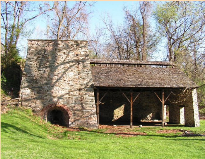
The reconstructed casting shed at the Catoctin Furnace. Here molten iron would have been poured into “pig-iron” molds.
