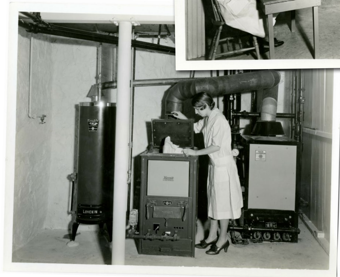
A Kernet gas fired incinerator next to a gas boiler
