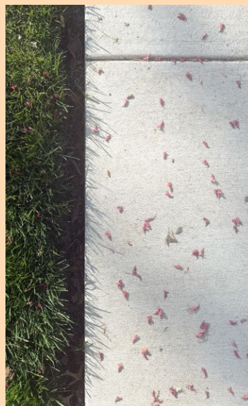
Sidewalk repairs in Guilford must utilize an exposed aggregate finish. The image above shows an original section of sidewalk, while the image at left shows a recent repair that does not meet the required standard.
